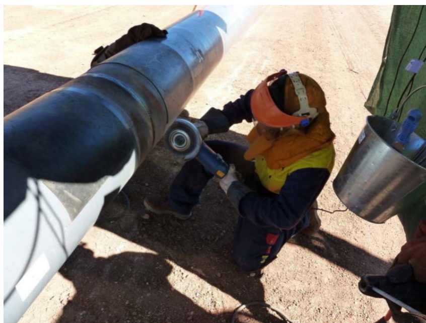
Figure 1: Operator buffing underside of pipe weld.
