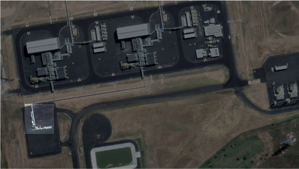
Figure 7: Orana Gas Processing Facility Custody Transfer Metering Facility 7
