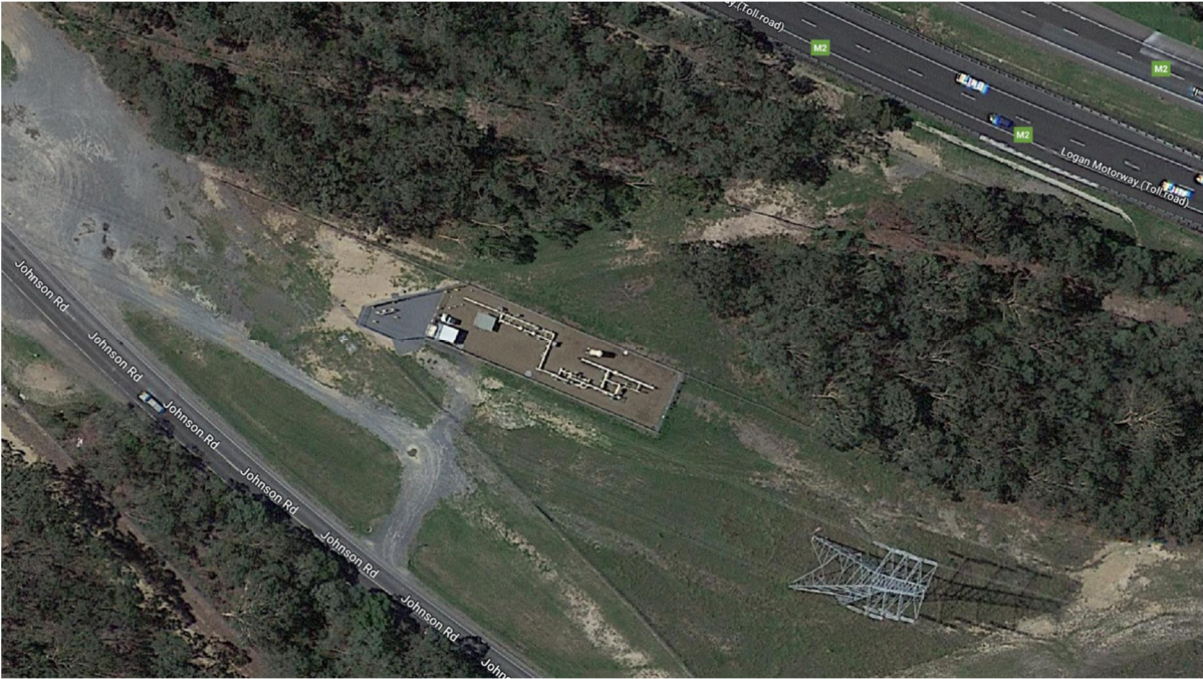
Figure 5: Ellengrove Gate Station on the Roma to Brisbane Pipeline 7
