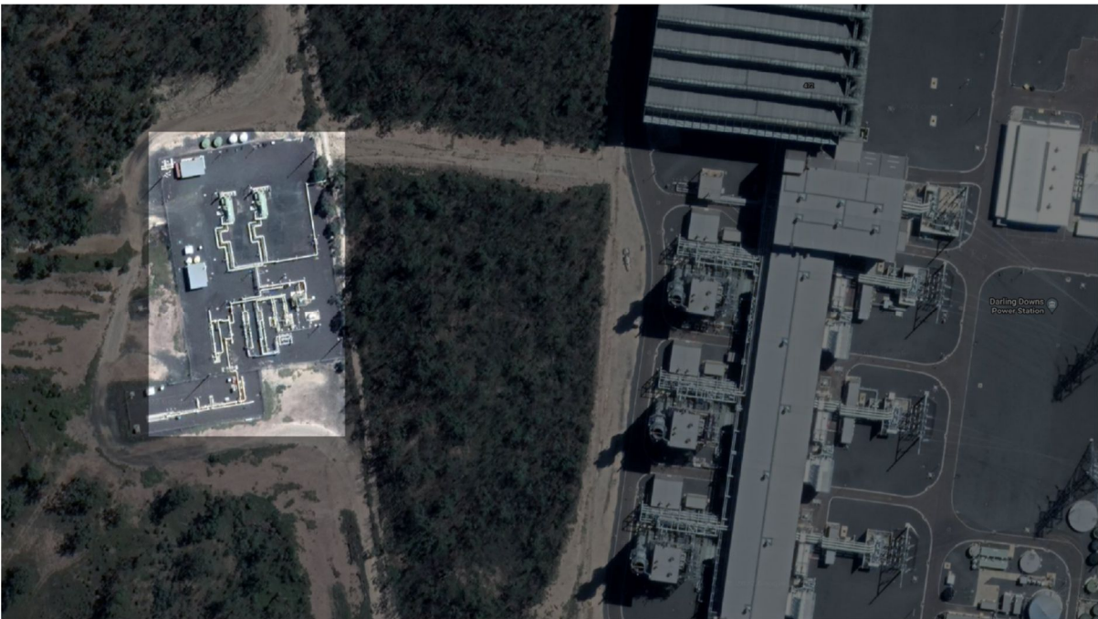
Figure 6: Darling Downs Power Station Custody Transfer Meter Station 7
